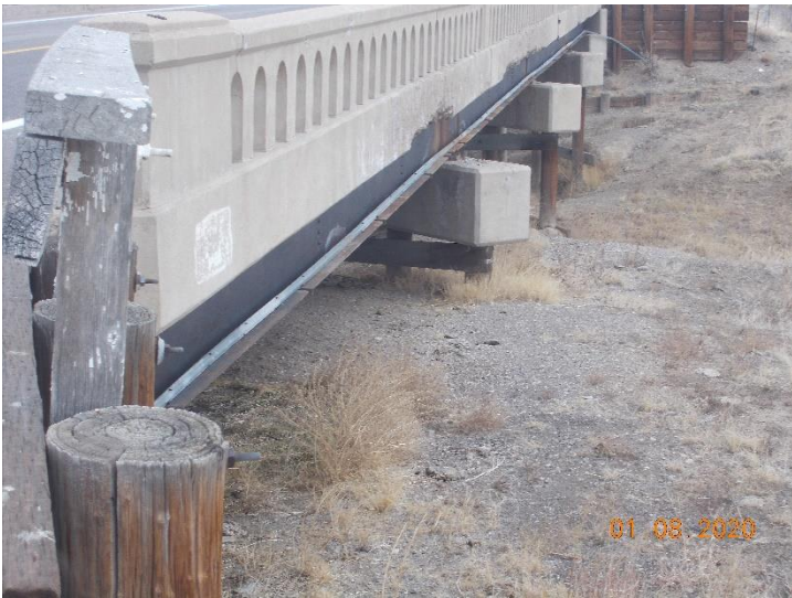
Paint sample N-21-F-LP02. The black paint is considered lead-based paint.
