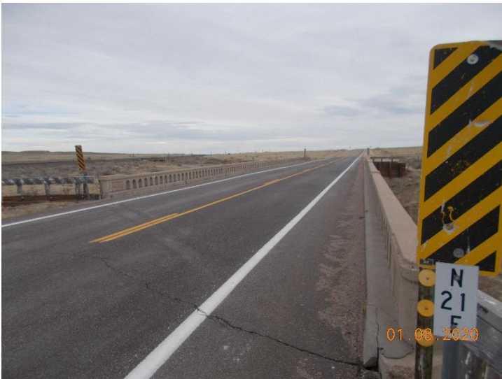
View of bridge N-21-F looking northeast.
